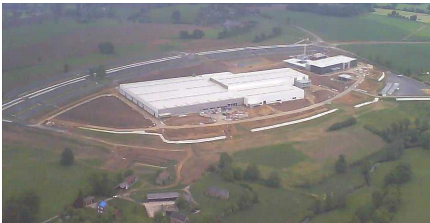
Faurecia Caligny site under construction [1]
